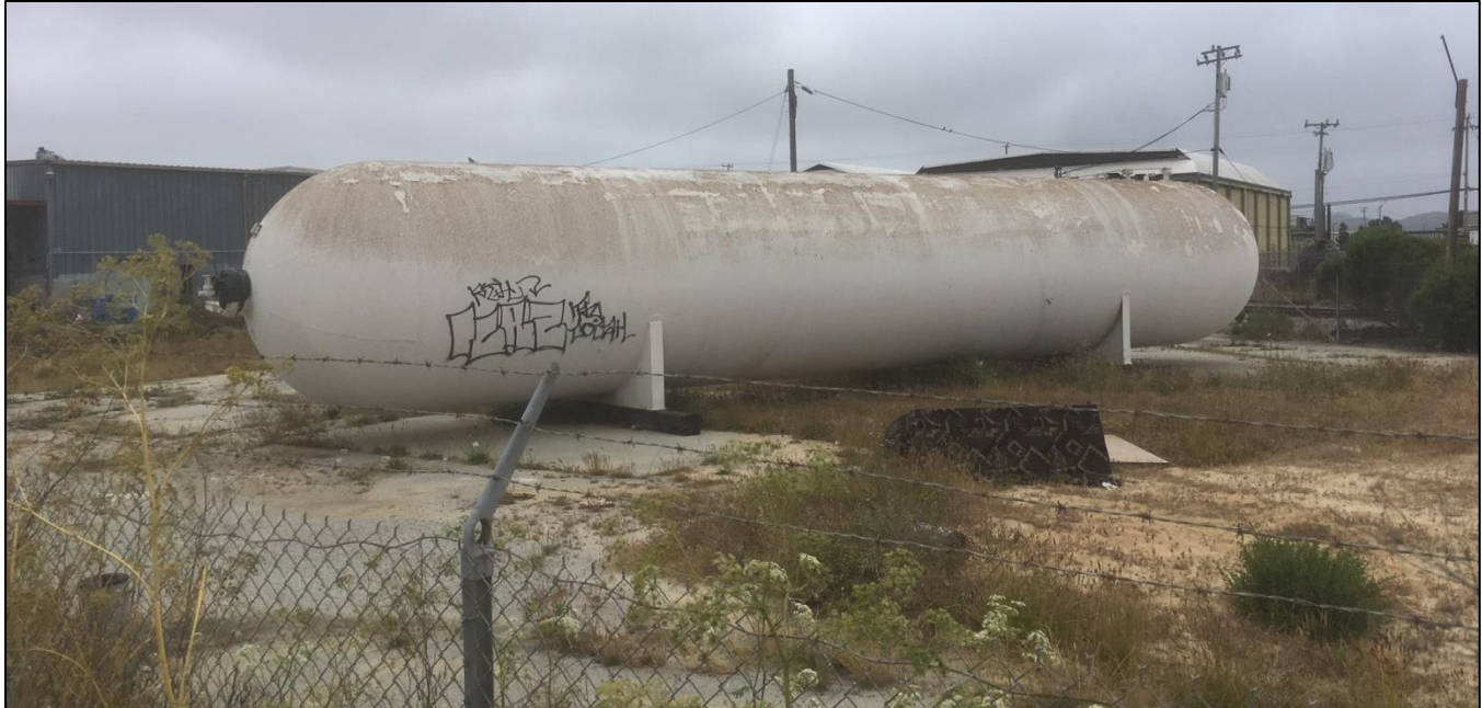
FIGURE 1 Photograph of storage tank on the subject site
